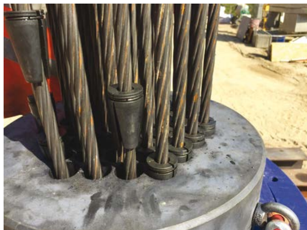
Picture 7.19a: Wedges being positioned (© Soletanche Bachy)
