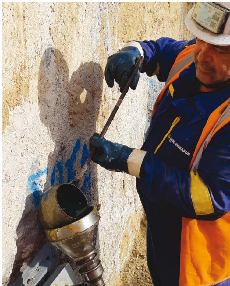
Picture 6.5: filling a trumpet tube with anti-corrosion product (wax)
