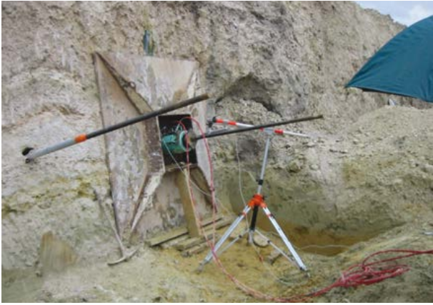
Picture 8.1b: steel reaction mass for a failure test (© Spie Fondations)
