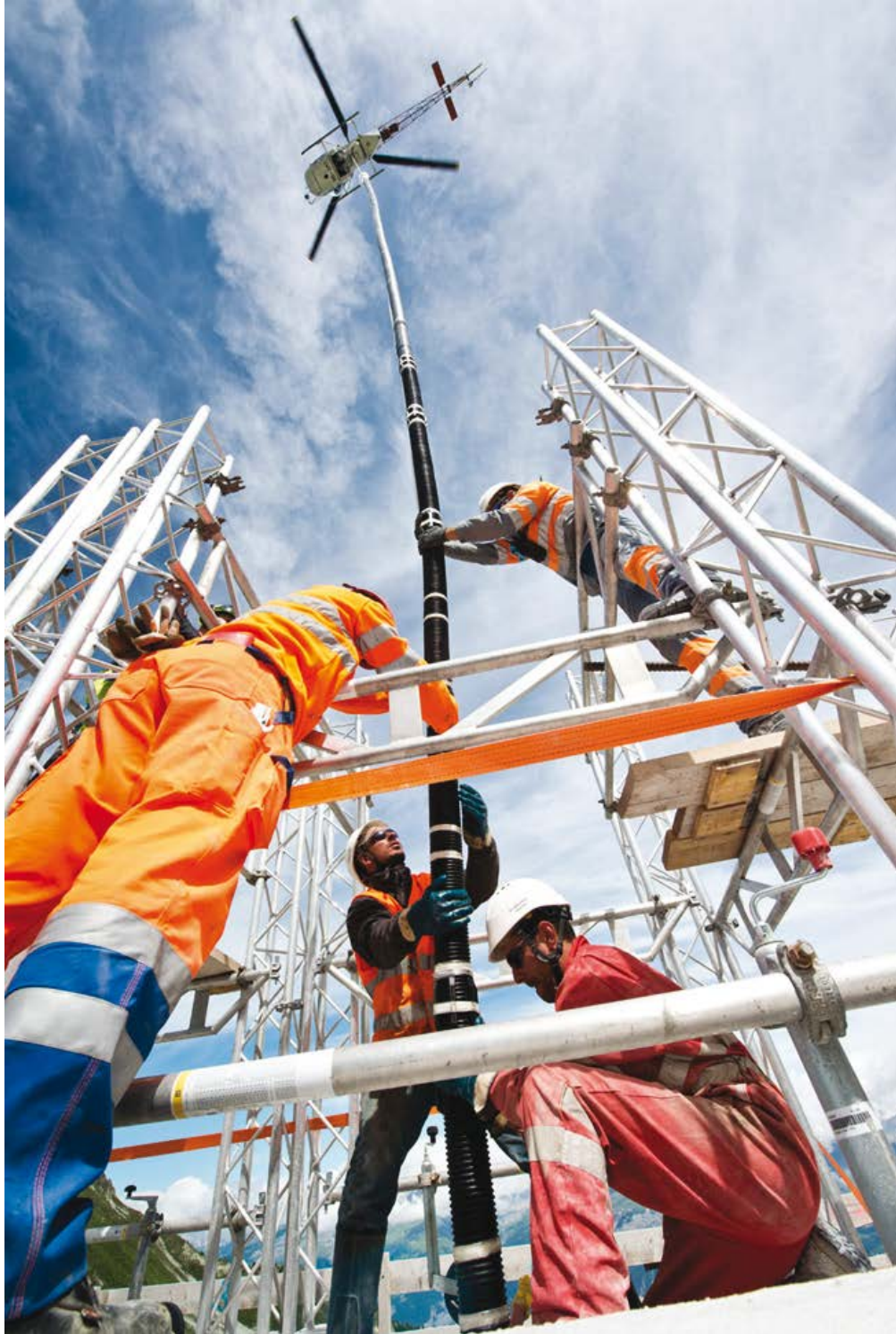
Picture 7.9: installation via helicopter (©Cédric Helsy- Soletanche Bachy)
