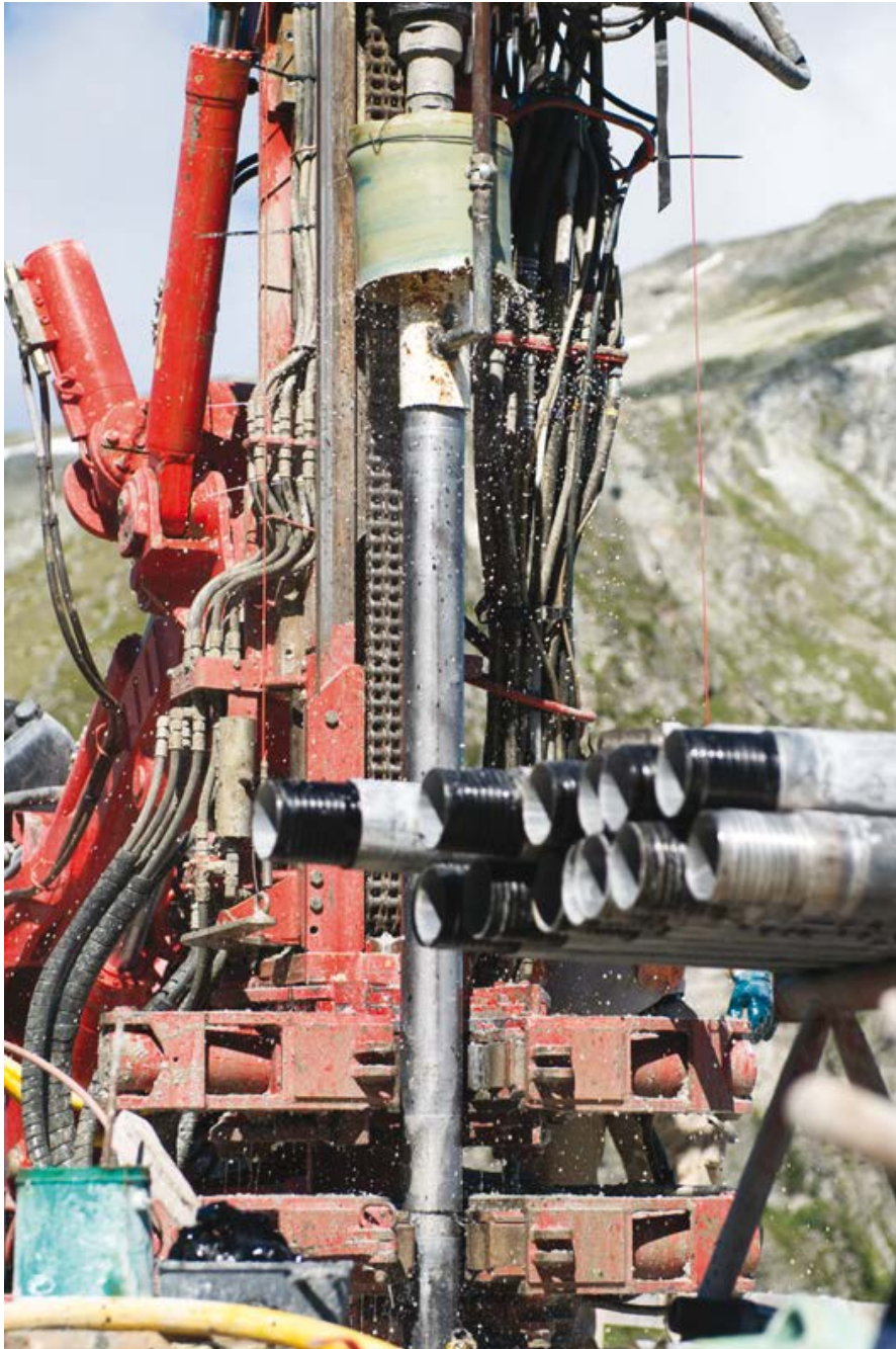
Picture 7.5: drilling rig in action (© Cédric Helsy- Soletanche Bachy)
