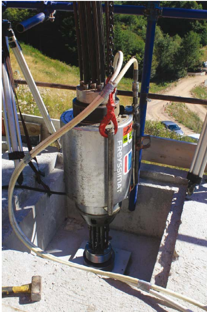
Picture I.4: example of a stressing jack (© Freyssinet)
