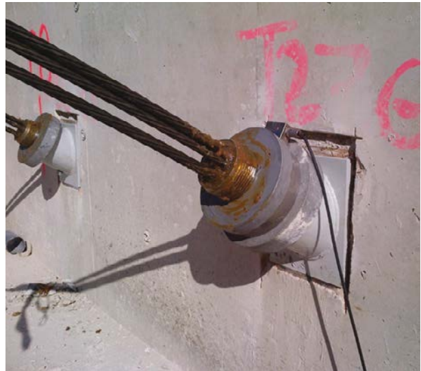
Picture 8.5: instrumented anchor head (© Freyssinet)
