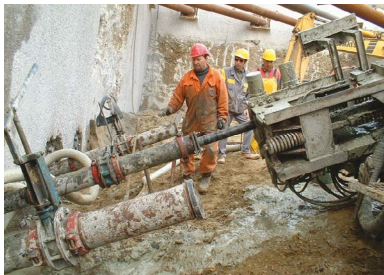
Picture 7.6: borehole under water-lock (© Sefi Intrafor)
