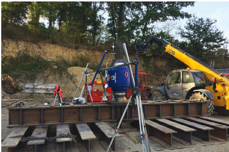
Picture I.1: Support structure for a loading test (© Soletanche Bachy)
