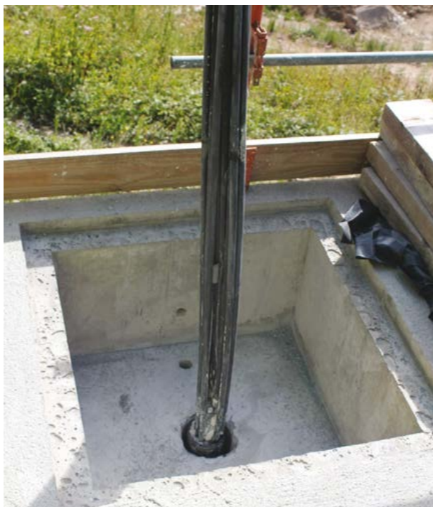
Picture 4.2: Outfitting a recess on a dam crest (© Freyssinet)
