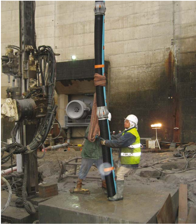
Picture 4.3: centralizers (grey) and tubes à manchettes (blue) (© Spie Fondations)
