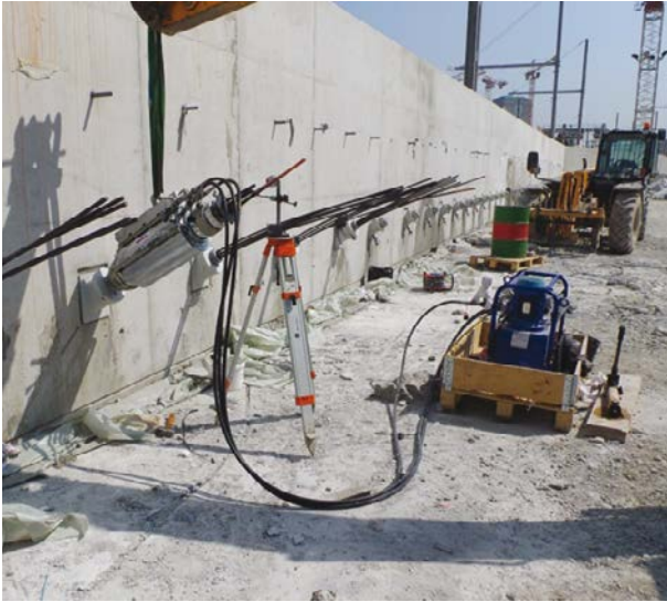
Picture 8.4: suitability test (© Soletanche Bachy)
