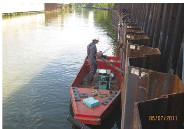
Picture 7.17: Example of ground anchor stressing on a sheet piles wall
