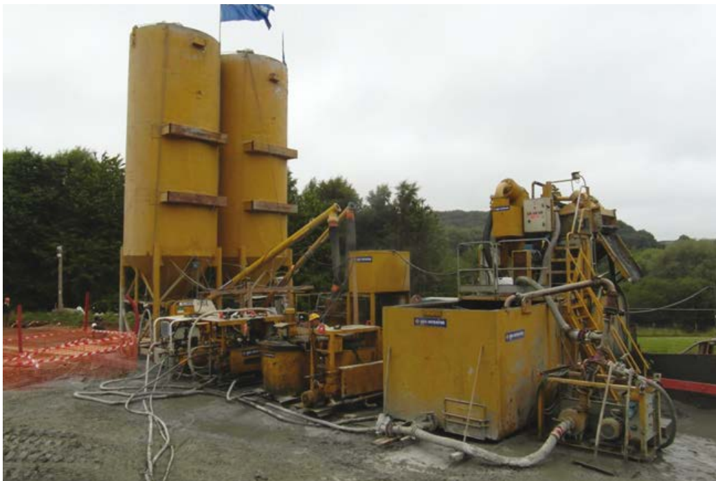
Picture 7.11: grout manufacturing unit (© Sefi Intrafor)
