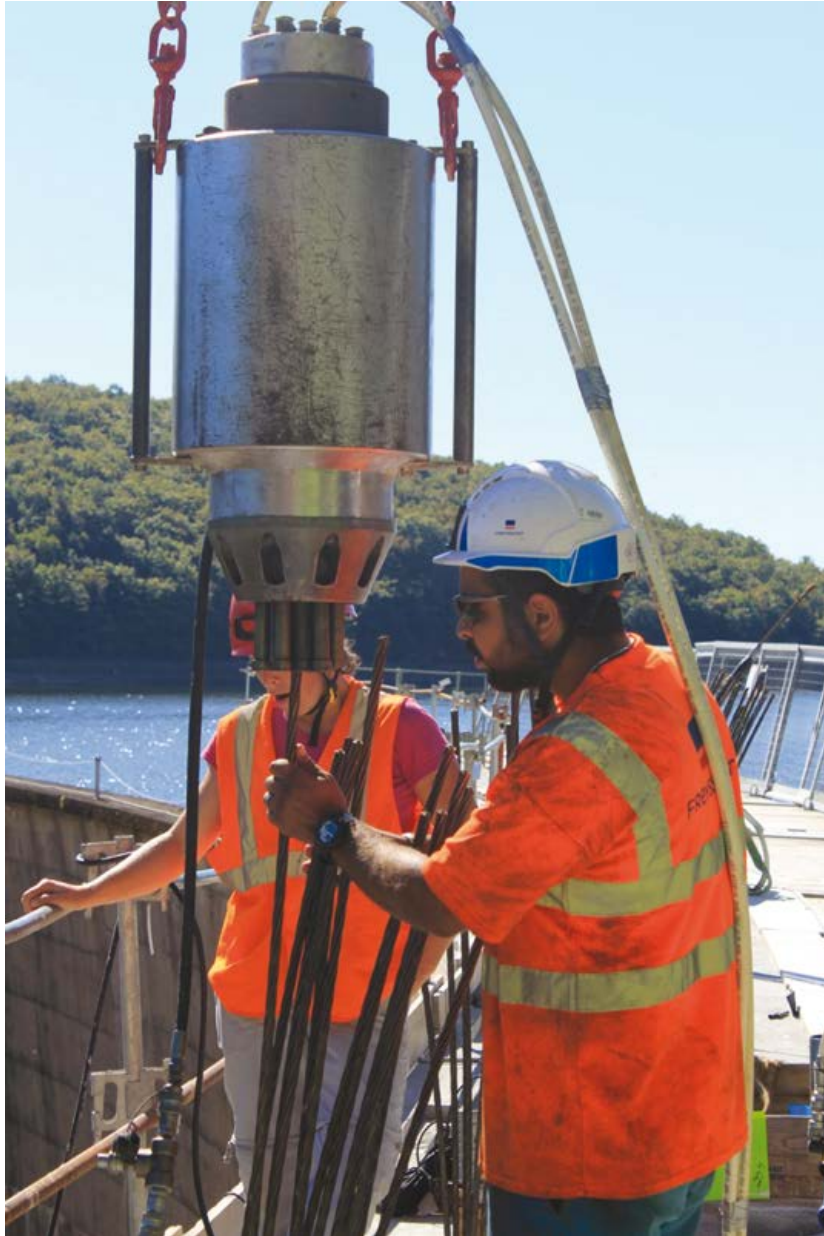
Picture 7.16: Installation of the stressing jack on a strand ground anchor (© Freyssinet)
