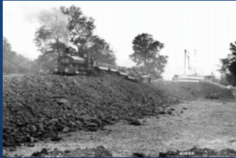
Deep Seated Delayed Failure of Railway Embankment (6m high Grass Covered Slope)
