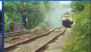
Track Deformation. Seasonal Movement of Railway Embankment (Mature Tree Covered Slope)
