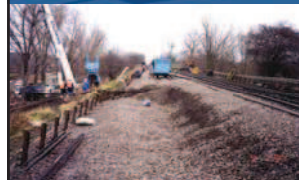
Deep Seated Delayed Failure of Railway Embankment (6m high Grass Covered Slope)
