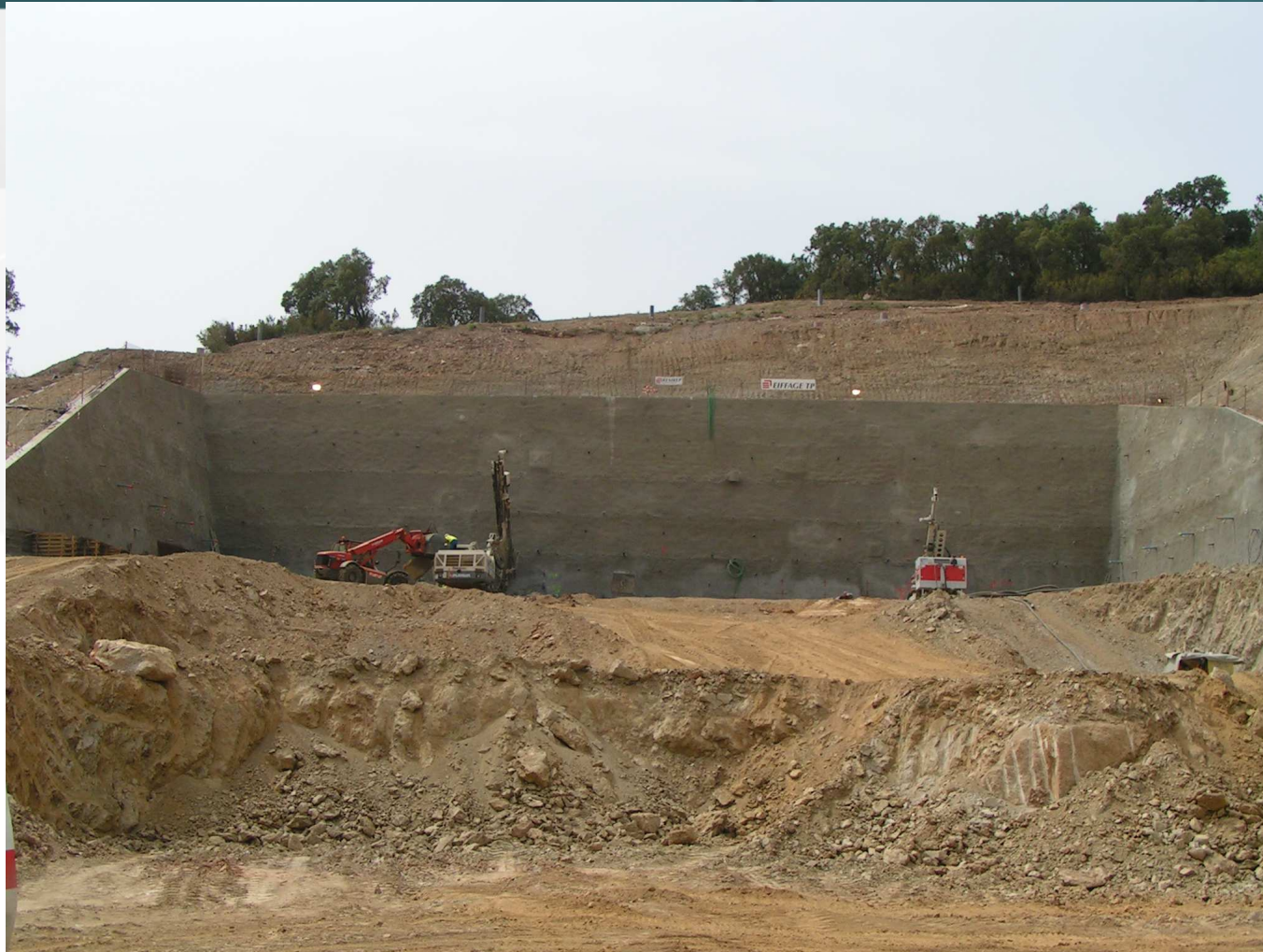
General view at the Northern head of the tunnel (excavation = 40 %)
