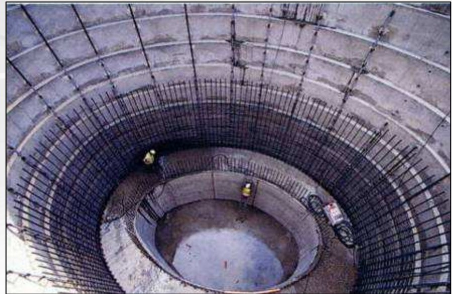
Concreting of a borehole
