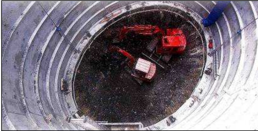
Excavation with BA concrete supports
