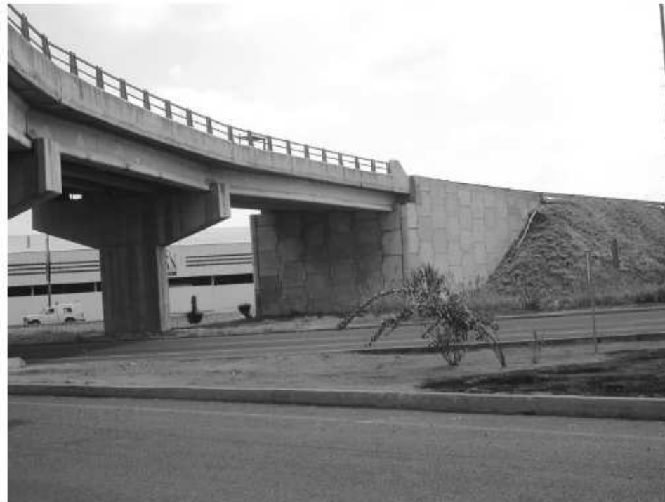
Figure 19. Southeast and front MSE wall of Bridge 1 at multiple interchange located along Highway 200 near Tecomán (N18.94442, W103.89845).
