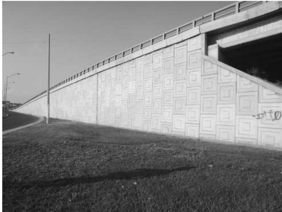
Figure 18. Well-performing MSE wall located near the entrance to the Port of Manzanillo (N19.07856, W104.28715).
