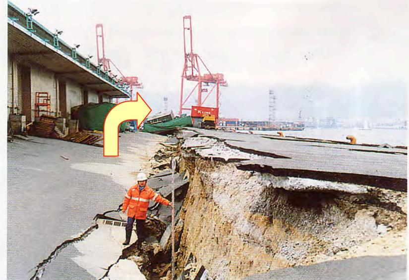
**Photo 11. Damaged caisson type quay walls at Port Island in Kobe Port**
