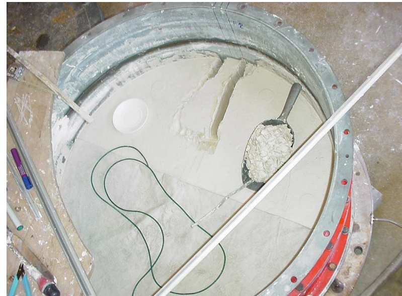
Installation of the pre-embedded anchors
