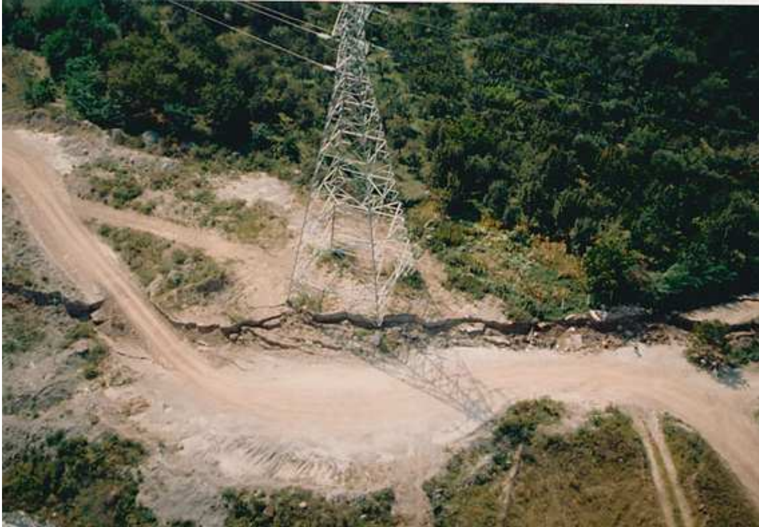
Thrust-faulting adjacent to an intact pylon (Golcuk)
