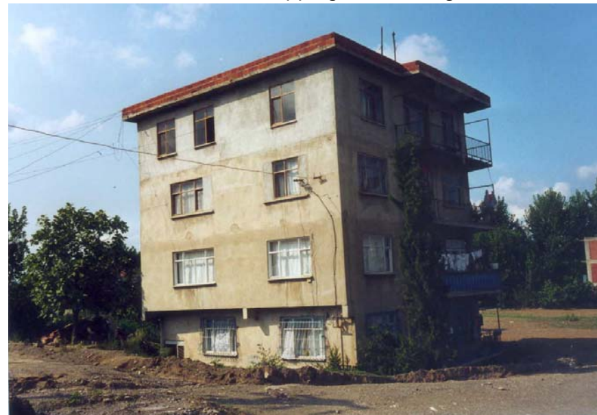
Building 1 : 4 storeys + Basement – No Damage
