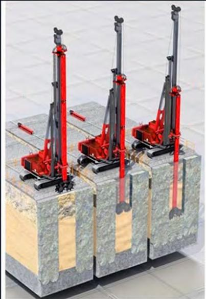
Cutter Soil Mixing technique
