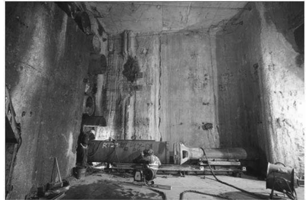
Figure 11. Setting up and welding – Beach Road rail tunnel.
