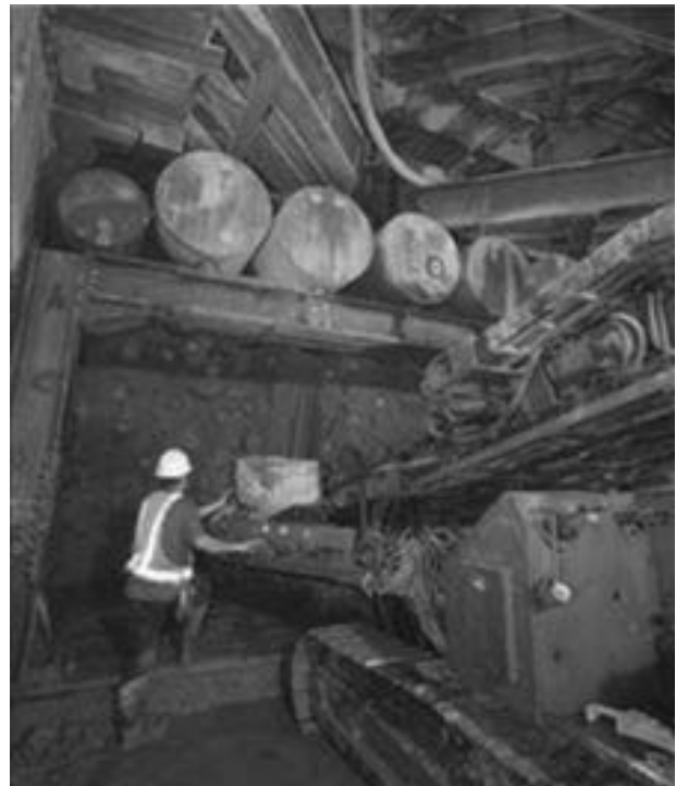
Figure 15. Drilling in the soil nails using the Springsol.
