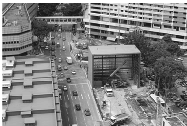
Figure 5. The acoustic enclosure around the top down access shaft adjacent to the Rochor Centre.
