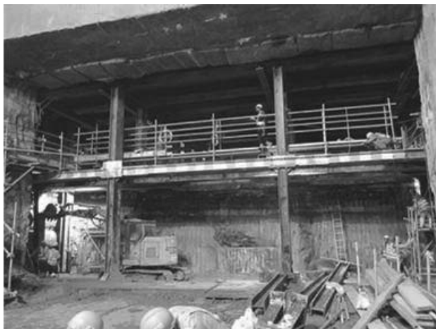
Figure 17. Central mining invert— Excavation and frames installation.
