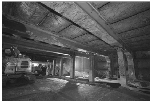
Figure 18. North Wing top heading -Roof pipes and heavy frames.
