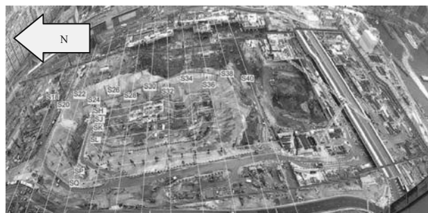
Figure 1. Deep excavation at West Kowloon Terminus (WKT).
