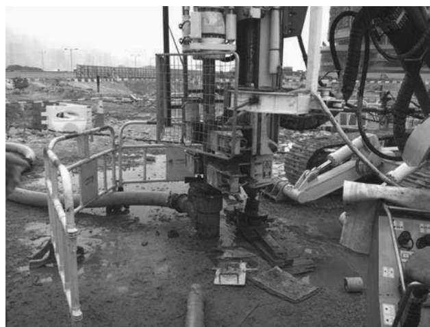
Figure 5. Plant used for jet grouting works with fully automated control system.
