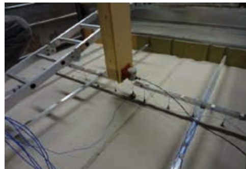
Figure 6. Measurement configuration for the concrete barrier test.
