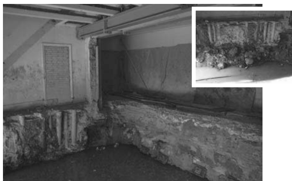
Figure 1. Indoor wet excavation.
