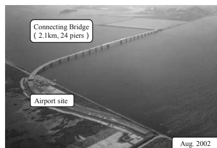
Figure 1. Overview of connecting bridge under construction
