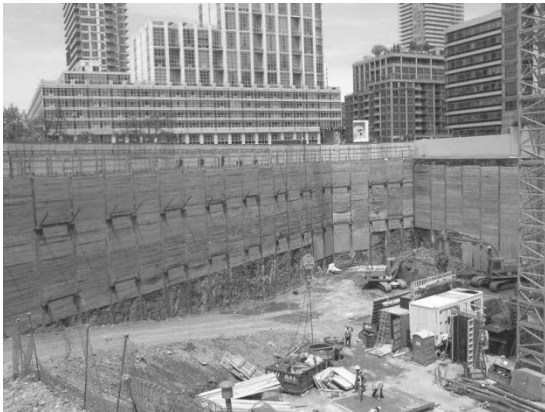
Figure 1. Outlook of soldier piles with wood lagging supported by tiebacks
