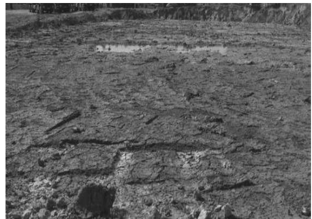
Figure 3. The view of the typical system of clays in the gout of the large building excavation with extremely diverse proprieties, simultaneous drying - the nearer zone, and irrigating - the background.
