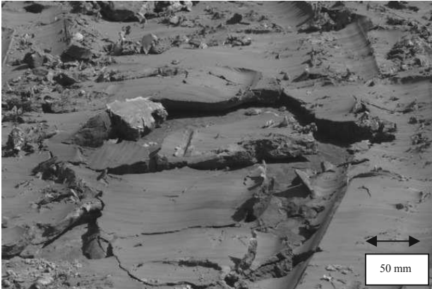
Figure 5. The natural process of clay drying after exposure of the excavation's bottom, (after 2 hours) the superficial macrodisintegration fully developed.
