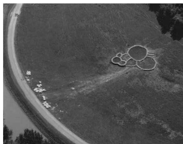
Figure 3. Piping (soil boiling) far away from the dyke, and stabilizing measures to reduce the hydraulic gradient (photo: L. Nagy).
