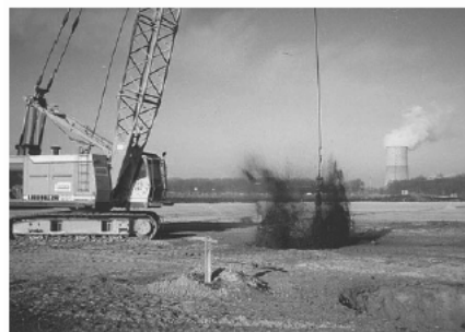
Figure 2. Compaction of deposited waste by dynamic consolidation
