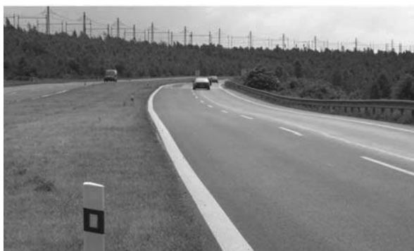
Figure 9. Photo of the top of Ervenice corridor
