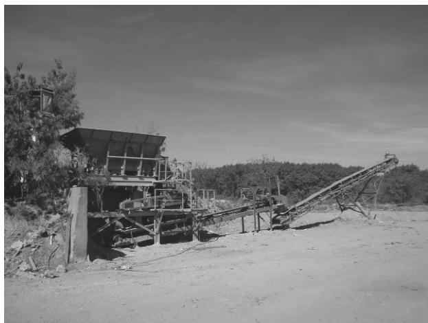
Figure 1. CDW Recycling Plant of Brasilia-DF.
