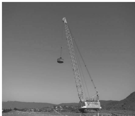
Figure 2. Dynamic Compaction Equipment.
