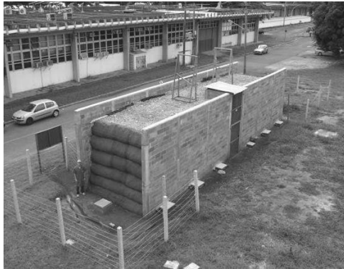
Figure 4. UnB retaining wall test facility (Figure 3 of Santos et al.).
