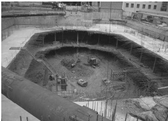
Fig. 4. Construction of parking by the method «UP-DOWN»
