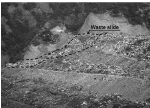
Figure 2. Waste slide view from the western side of the MSW landfill.
