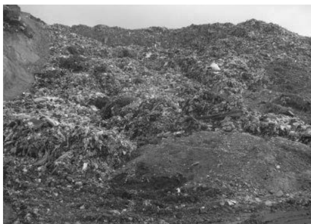
Figure 3. Waste slide view from the access bench located at the toe of the slide.
