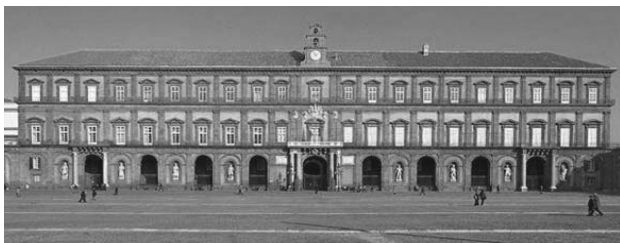
Figure 3. The Royal Palace of Napoli, built in the 17 th century, whose façade was modified blinding some of the arches in the 18 th century by architect Luigi Vanvitelli. Statues were added in the blinded arches in 1888.
