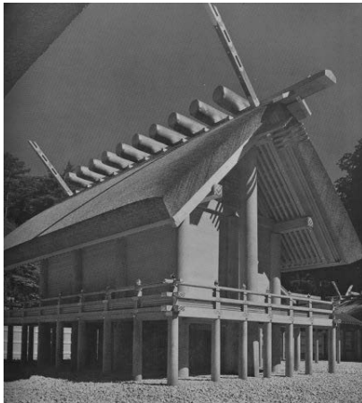
Figure 1. Ise shrine, which undergoes ritual reconstruction every 20 years ever since the 7 th century.
