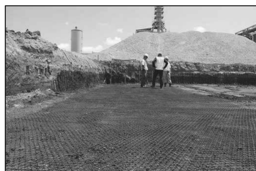
Figure 9. Laying of TriAx geogrids
