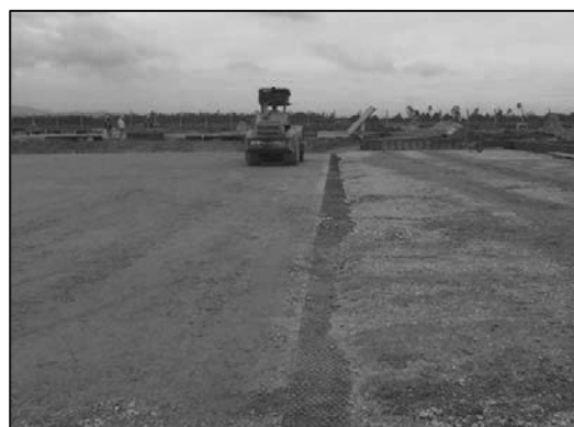
Figure 11. Construction of MSL with granular materials.
