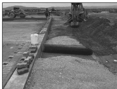
Figure 12. Placement of interlocking paving blocks.
