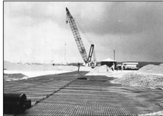
Figure 3. Platform rehabilitation work in progress. (after Yong, Chan et al., 1990)
