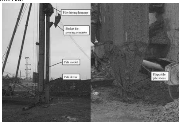
Figure 1. Physical diagrams of pile-driving machine: (a) XCC pile-driving equipment and pile mould; and (b) Pile driver locating and flappable pile shoes.
