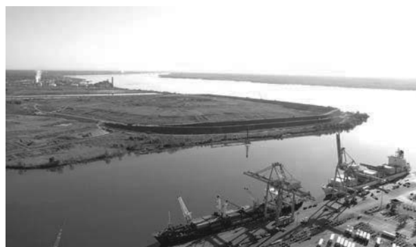
Figure 6. View of Completed MSE berm
