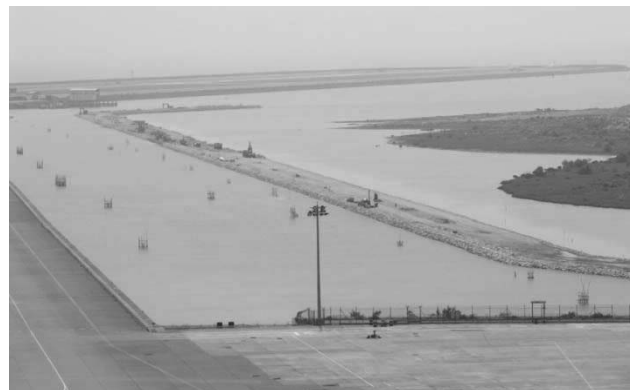
Figure 13. The Completed Stone Column Seawall
