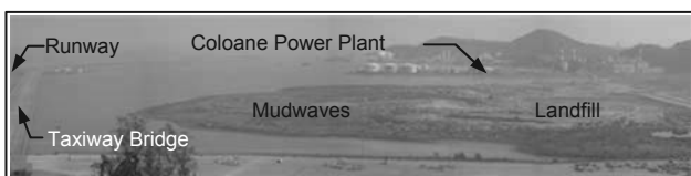
Figure 1. View of the Landfill Site and Mudwaves
