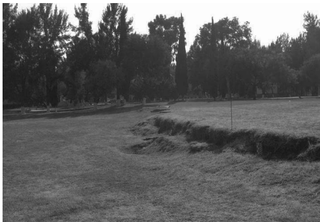
Figure 7. Crack in an abrupt transition area.
