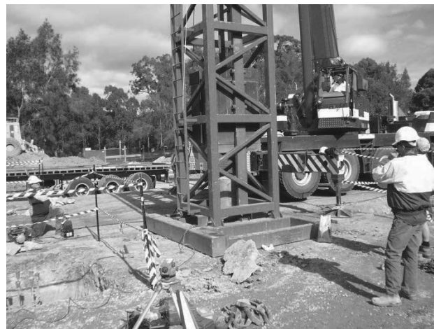
Figure 2. Dynamic pile load test set up in Case Study 1
