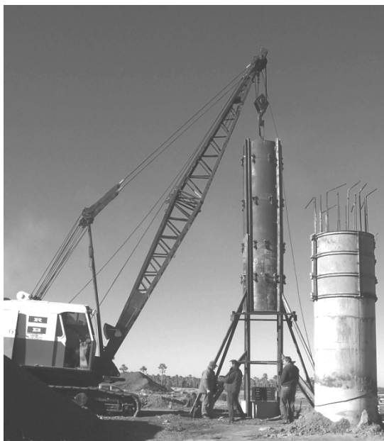
Figure 6. Picture of one of the piles tested at the site.
