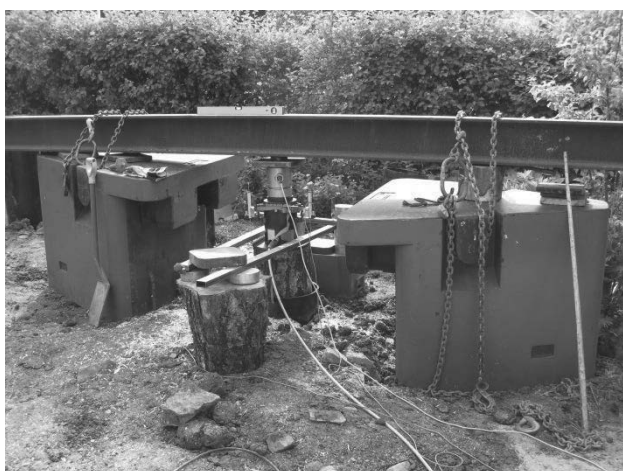
Picture 3. Arrangement of the load test in Turku 2010.
