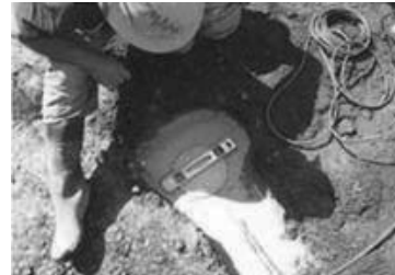
Figure 2. Installation of pressure cells below the footing-column unit.
