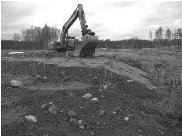
Figure 5 Construction up to height 1.5 m for embankment 1.
