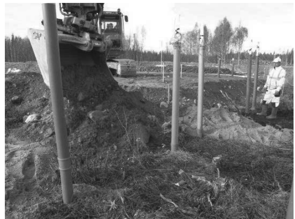
Figure 4 Cautious construction of embankment around the measuring equipment.
