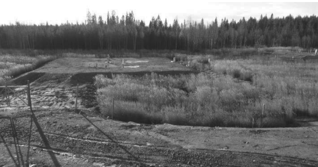
Figure 6 Finished construction of embankment 2 (1.5 m height). Photograph taken about two years after finished the construction.
