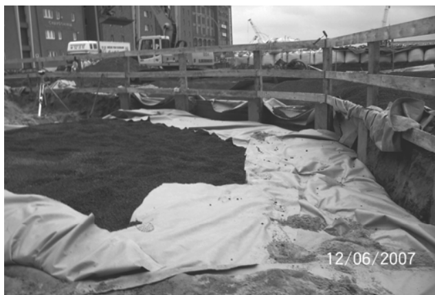
Figure 5: Placing of expanded clay
