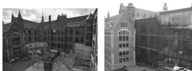
Figure 17. Finished outside construction
