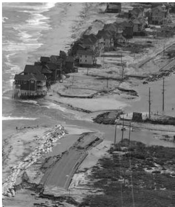
Figure 1. A section of Highway 12 at the edge of Rodanthe, N.C. undermined by erosion due to the storm surge and wave action during Hurricane Irene. (Photo: News & Observer, Aug. 31, 2011)
