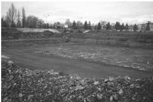
Figure 1. Excavation pit on a site
