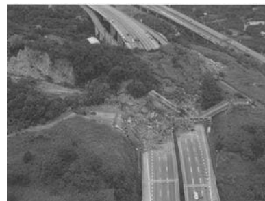
Figure 1. National Highway No. 3 at 3.1k accident
