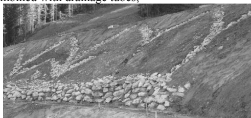
Figure 3: reservoir slope featuring drainage trenches above the storage level.
