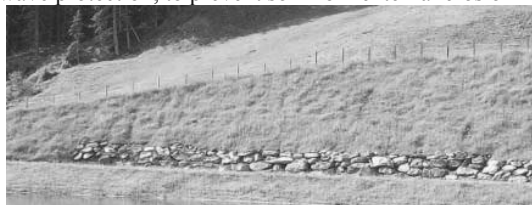
Figure 4: Wave protection measure (stone wall) in an impounded reservoir.
