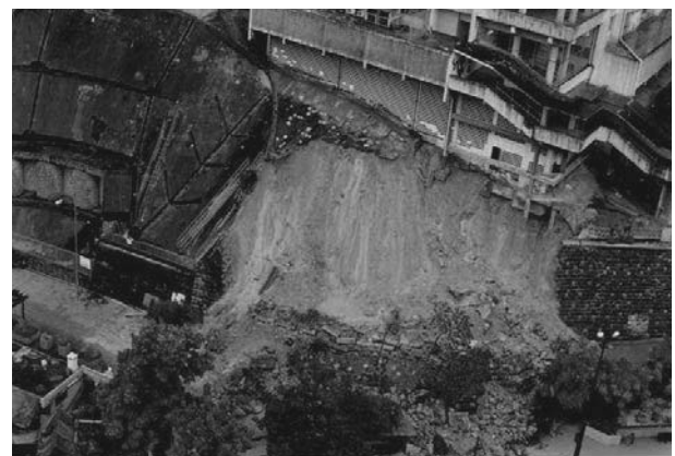
Figure 1: The Kwun Lung Lau Landslide in July 1994
