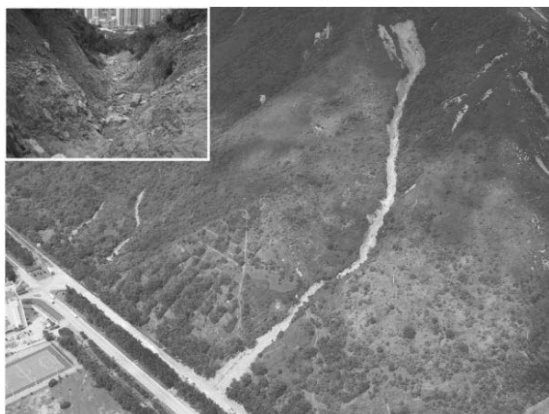
Figure 5: Yu Tung Road channelized debris flow
