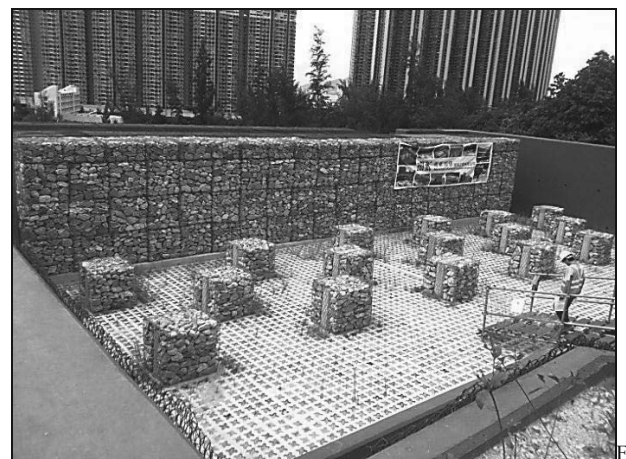
Figure 1. Array of baffles installed in front of a rigid barrier in Lantau Island, Hong Kong
