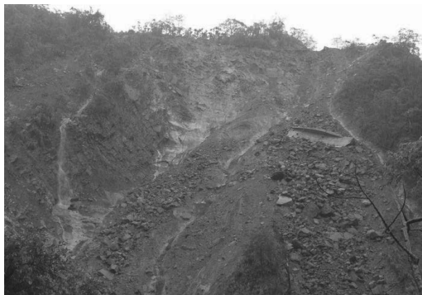
Figure 8. Failure of box-structure road section due to Typhoon Talim.
