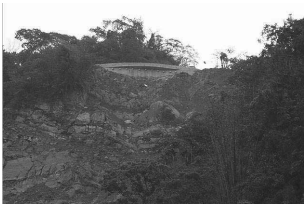
Figure 7. Completion of box-type structure at Mileage 39Km.
