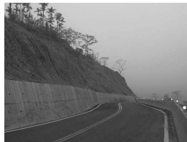
Figure 10. Completion of upslope remedial works at Mileage 39Km.
