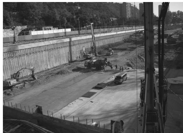
Figure 5. Foundation pit with dimensions of 265 x 53,5 m and depth of 12 m next to Danube river.
