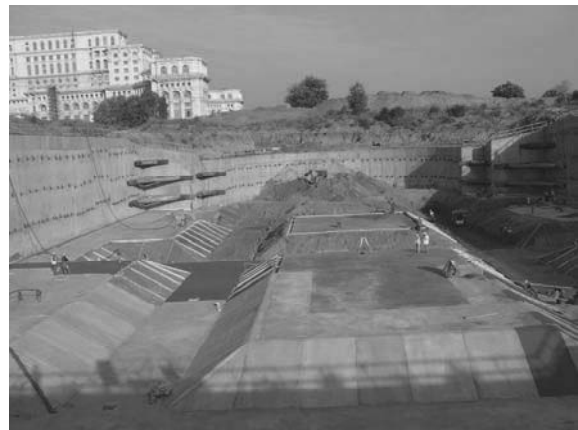
Figure 8. Final stage of excavation
