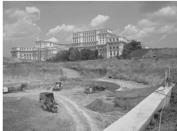
Figure 7. Installation of the first level of anchors
