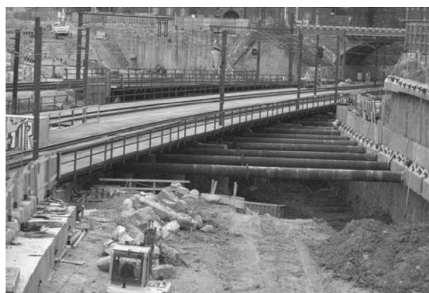
Figure 15. Picture of the railway crossing, December 2012.
