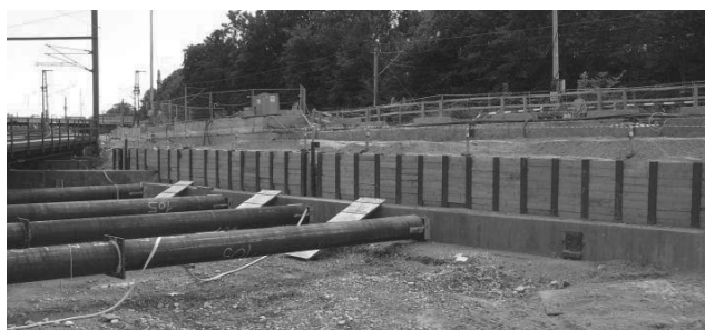
Figure 9. Encastered soldier pile wall.
