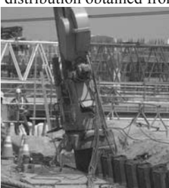
Photo 2. Overall view of installation work
