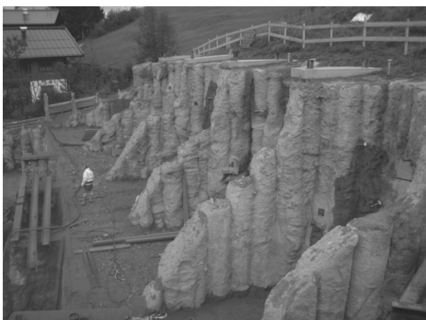
Figure 6. View of excavated MIP-walls
