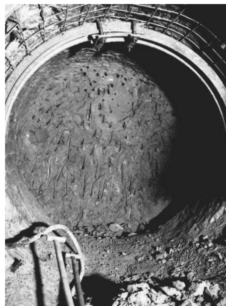
Figure 3. Circular adit used in backanalyses of the earth pressure coefficient at rest K_0 (Pavlík et al., 2004).
