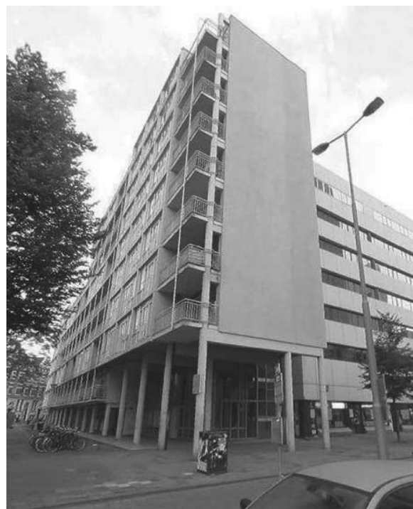
Figure 3. The apartment building.
