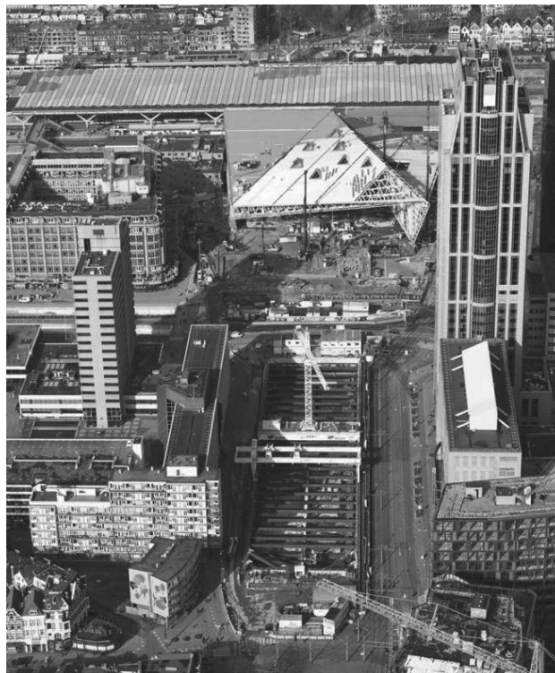
Figure 1. The construction of the underground car park Kruisplein (February 2012). The apartment building is situated in front, at the left (perpendicular to the car park). Photograph Nick de Jonge – Skeyes fotografie.
